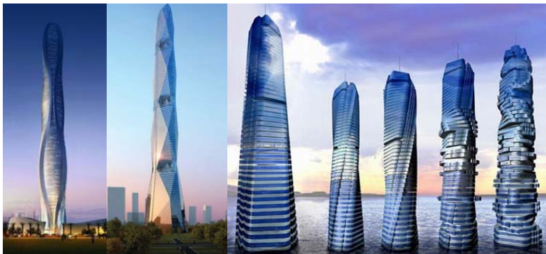
EP 07 Tower EP 15 Tower
