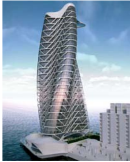
Strata Tower, Al Raha Beach Asymptote Architecture
